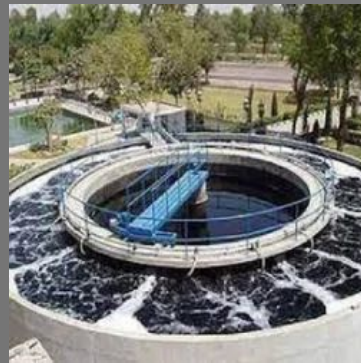
Effluent Treatment Plant
